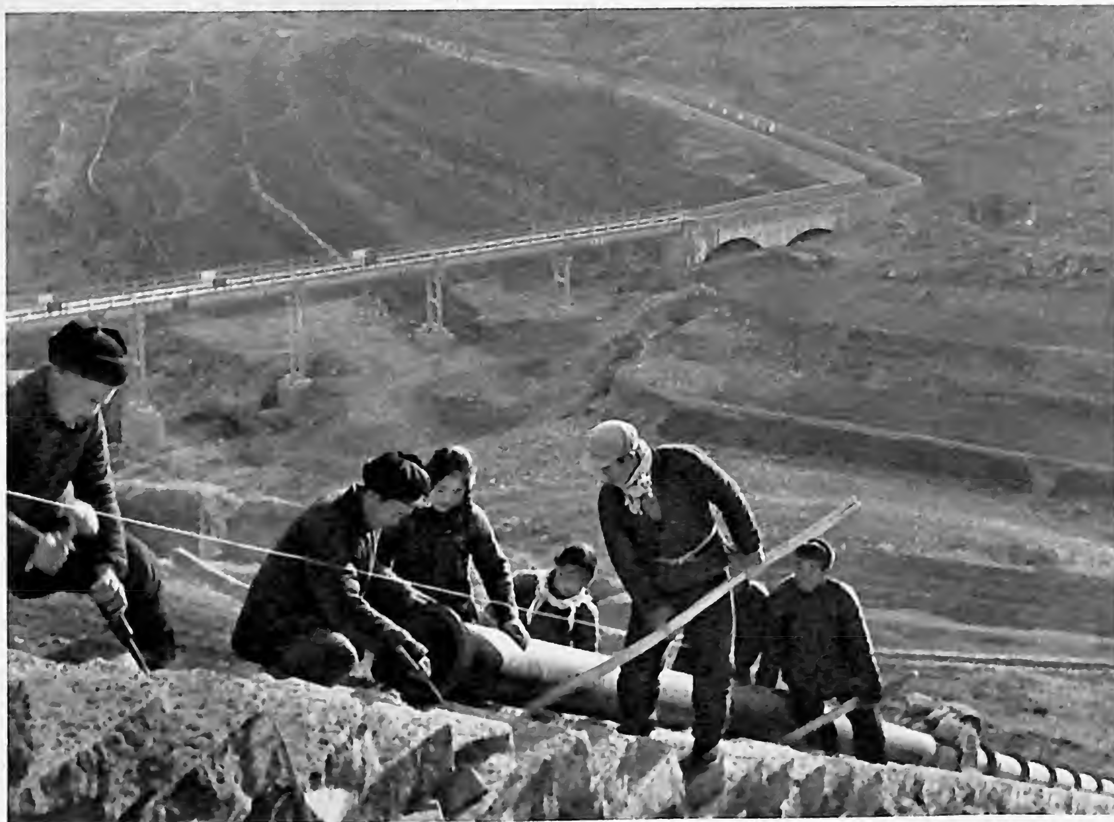
Commune members laying pipes for a pumping station in the Yintu brigade of Wuching commune, Linchu County, Shantung Province.
